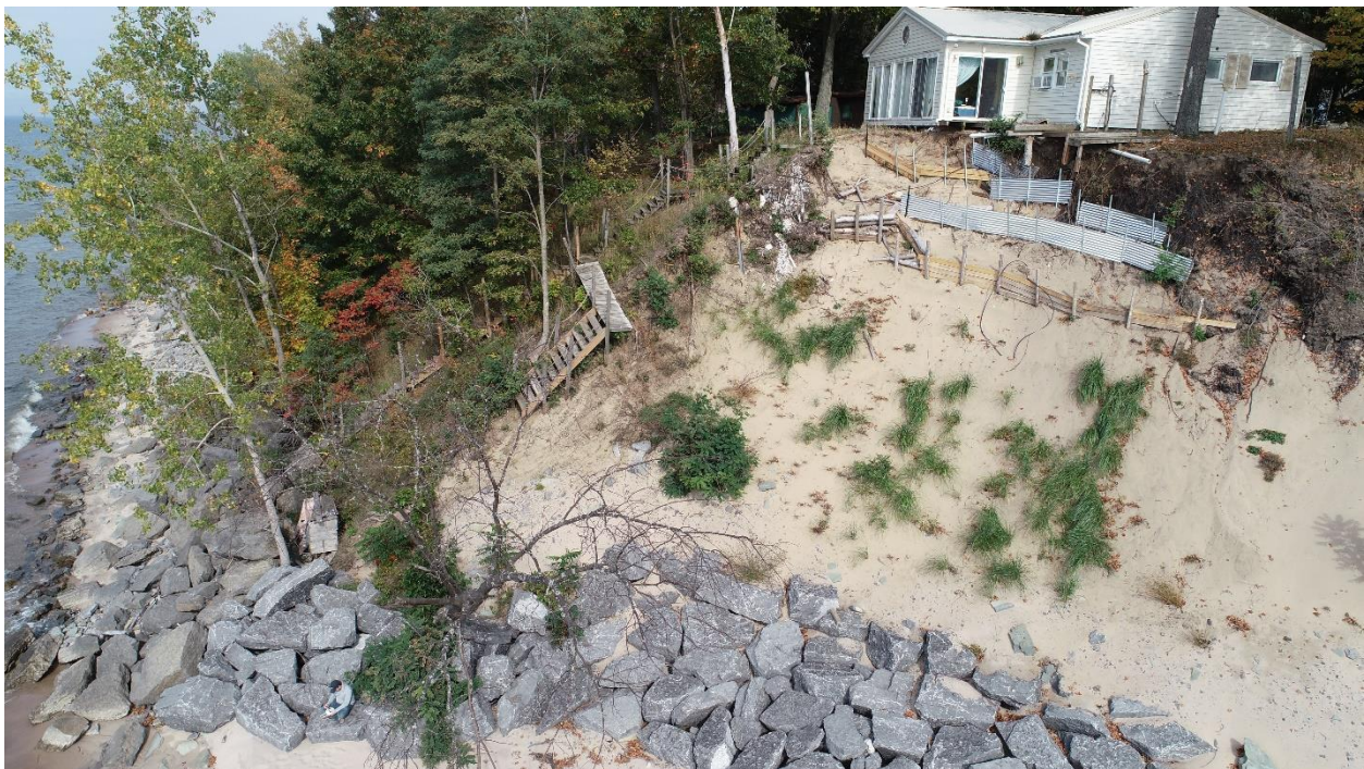
Figure 7. Limestone rip-rap and dune revegetation on display along the south spit, October 2021.
