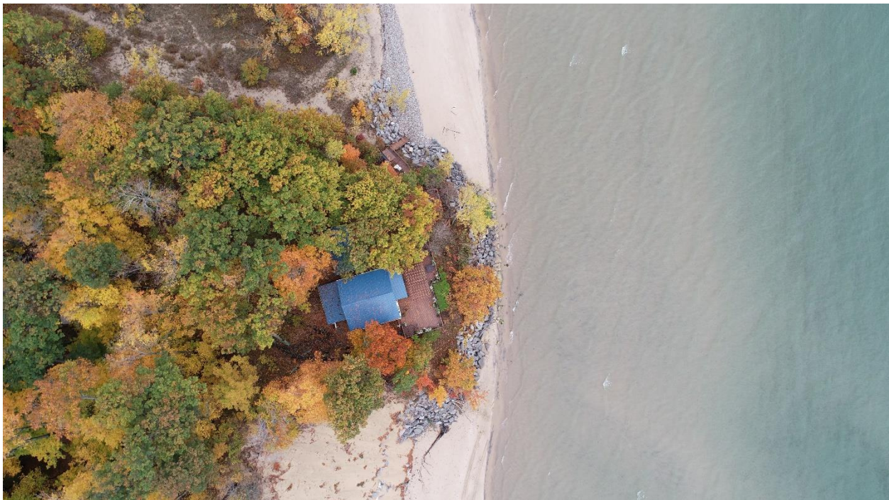
Figure 8. Headland created by artificial shoreline stabilization techniques, South Spit of Sandy Pond. Here, waves have been deflected away from the shoreline and into unprotected shoreline areas, resulting in additional, accelerated erosion along the flanks of the rip-rap wall.
